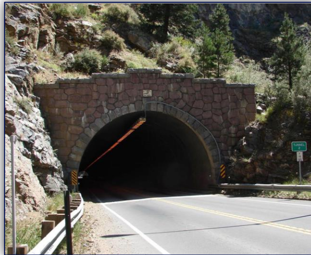
F-15-AX - US 6 Tunnel 2 in Jefferson County
