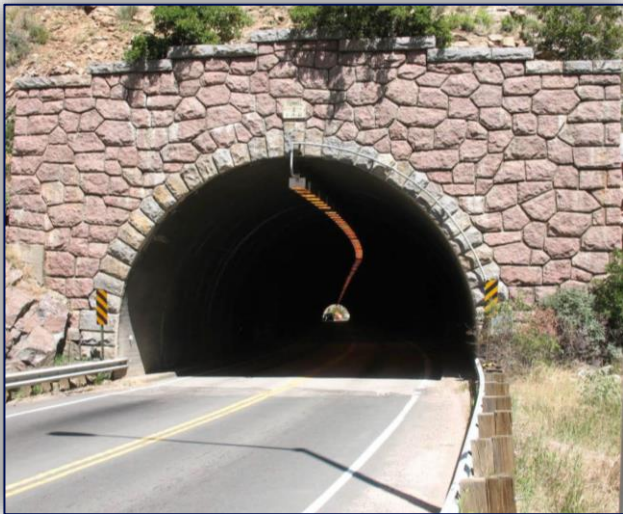
F-15-AY - US6 Tunnel 1 in Jefferson County
